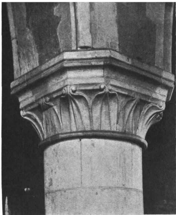
Detail of Nave Arcade.
